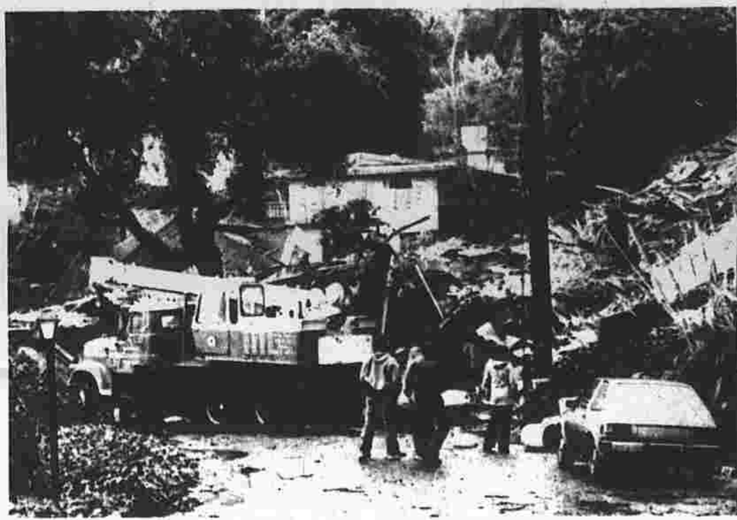
Neighbors view the rubble of one of two exclusive homes demolished by a massive mud slide, triggered by torrential rains, in San Rafael, Calif. Heavy equipment is being used to clear the street.
