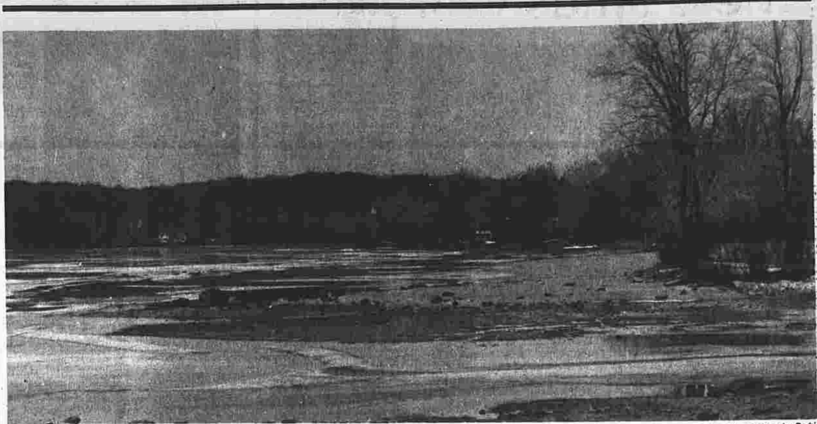
This is a view of Indian Notch Park and a portion of Bolton Lake from the dam. In the center is the old pier. The new erosion containing wall will run along the far side of it and further out into the water. On this side of the pier, and in the foreground, is some of the sand that has already escaped the beach area.
